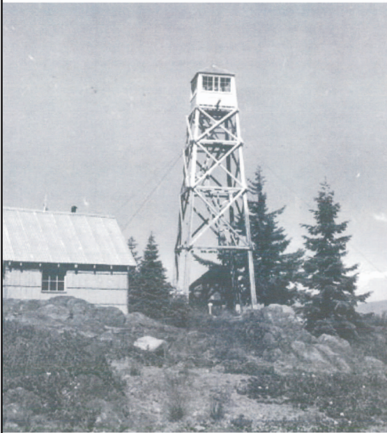
Communication tower disguised as a fire lookout tower.
